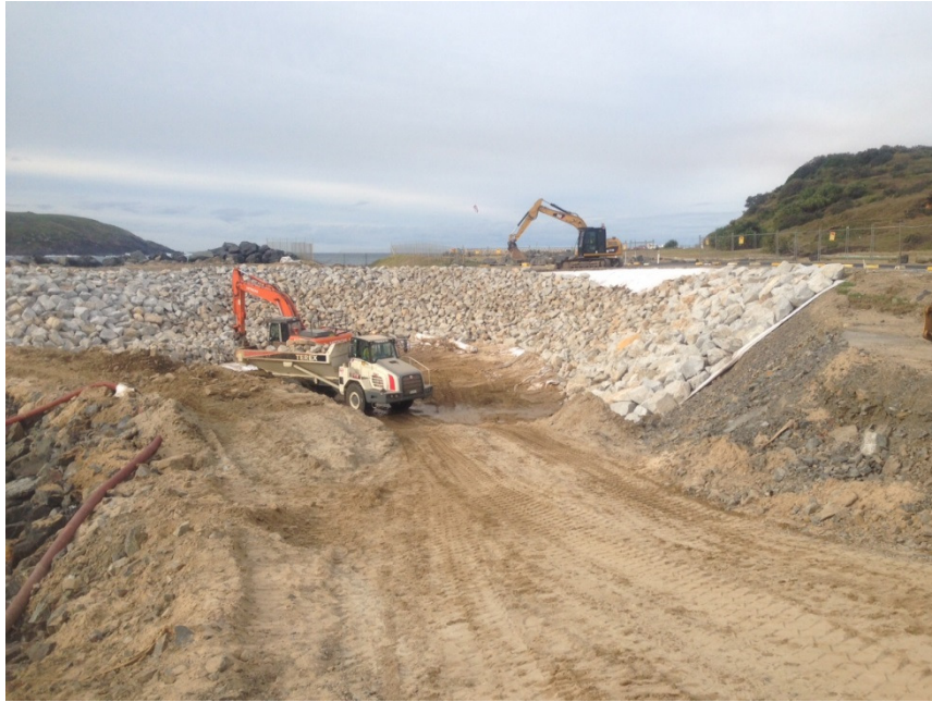
Photo 2 Construction in progress – 15 July 2015
