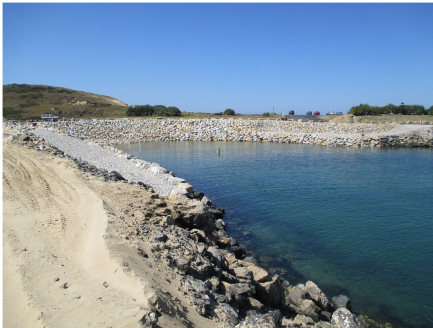
Photo 3 Completed basin extension – 3 October 2015
